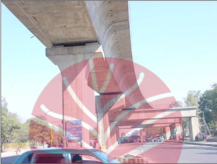
Fig. 3.2: Elevated Viaduct system
