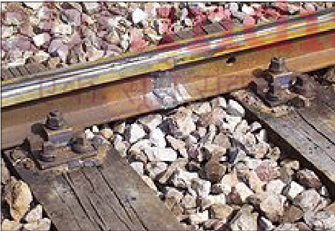
Fig. 3.5: Continuously welded rail.
